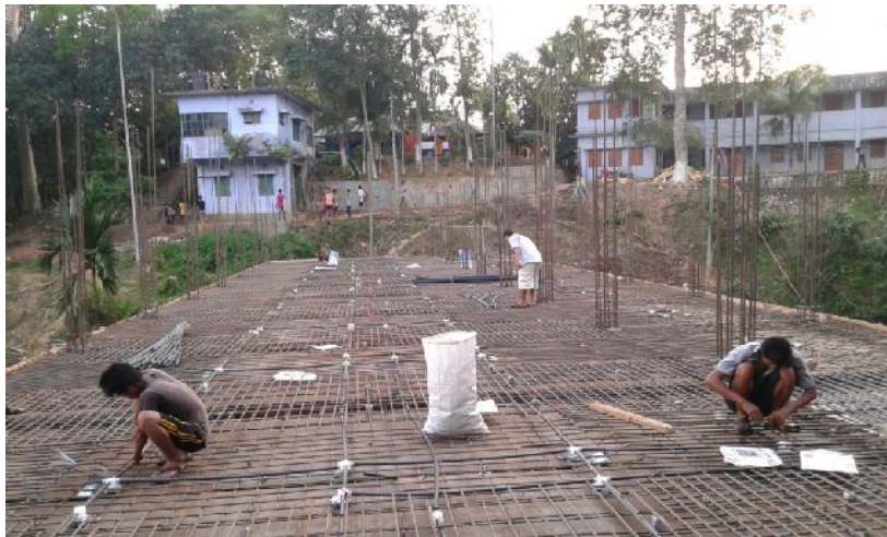
Plate 3: Fixing pipers for electrical lines
