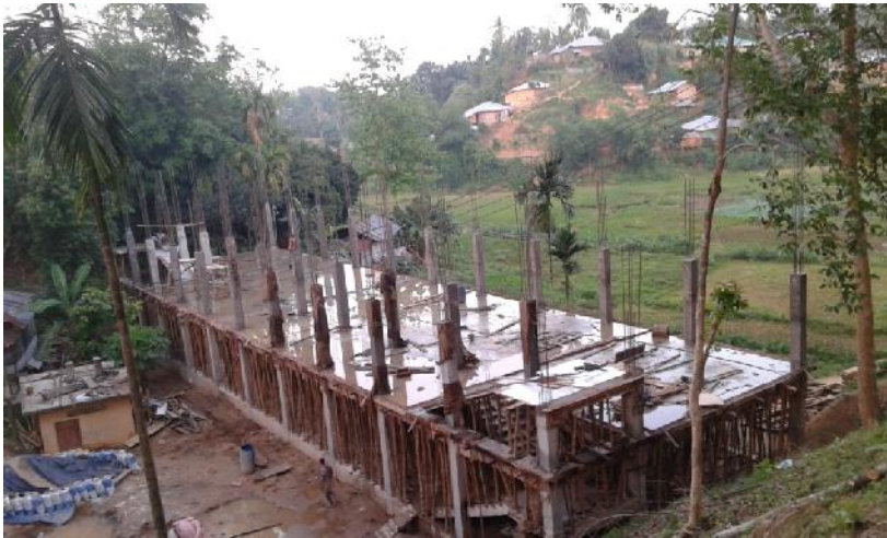
Plate 1: Building pillars for the 2 nd floor
