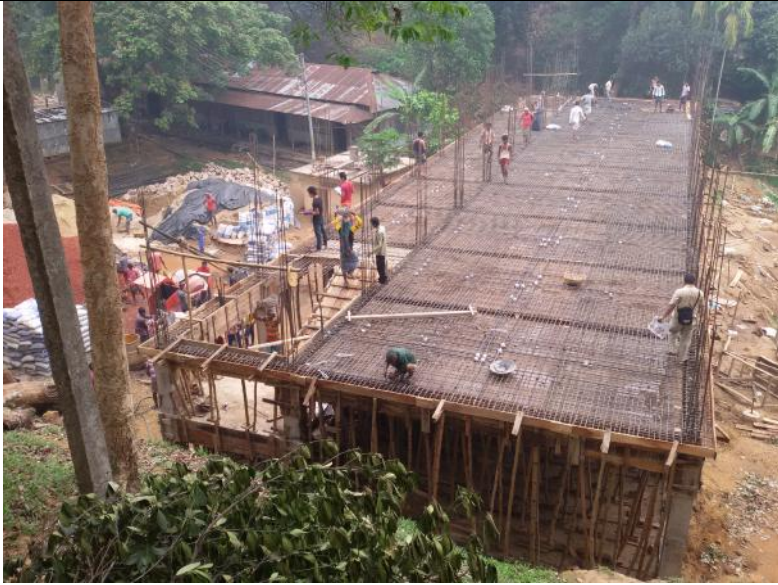
Plate 5: ready for casting
