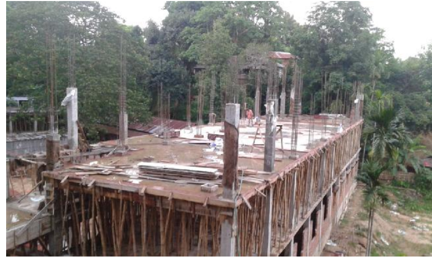
Plate 10: Putting up pillars for the 3 rd floor
