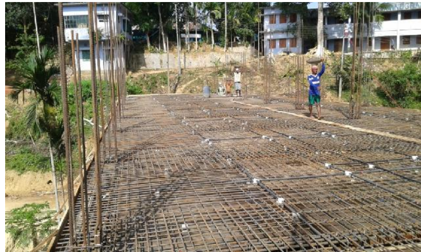
Plate 4: Ready for casting
