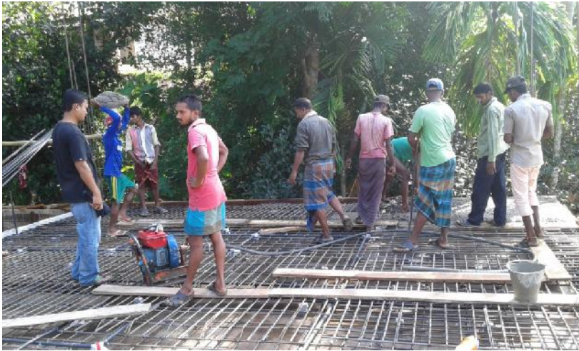
Plate 5: Casting on progress
