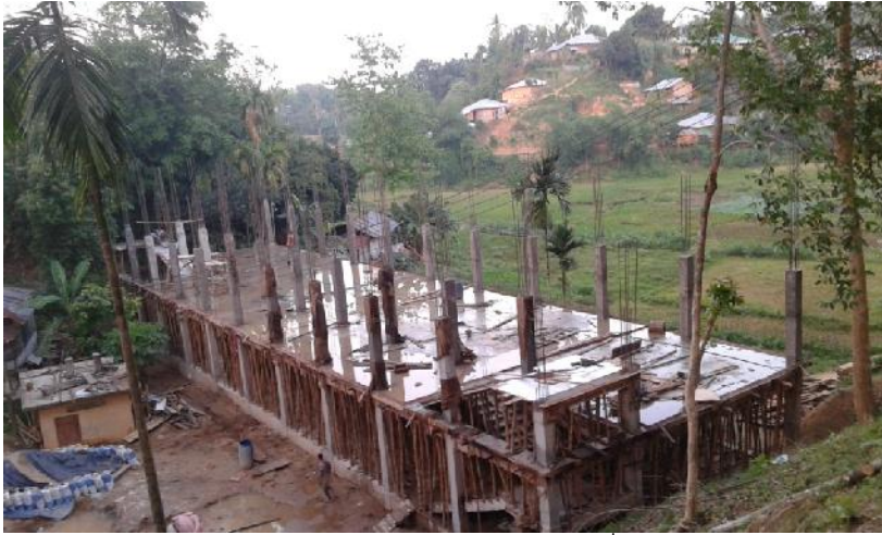
Plate 1: Building pillars for the 2 nd floor
