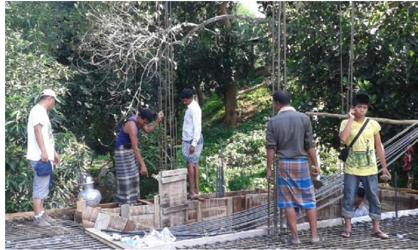
Plate 6: The engineer giving instruction to the mason
