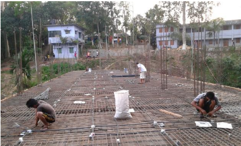
Plate 3: Fixing pipers for electrical lines
