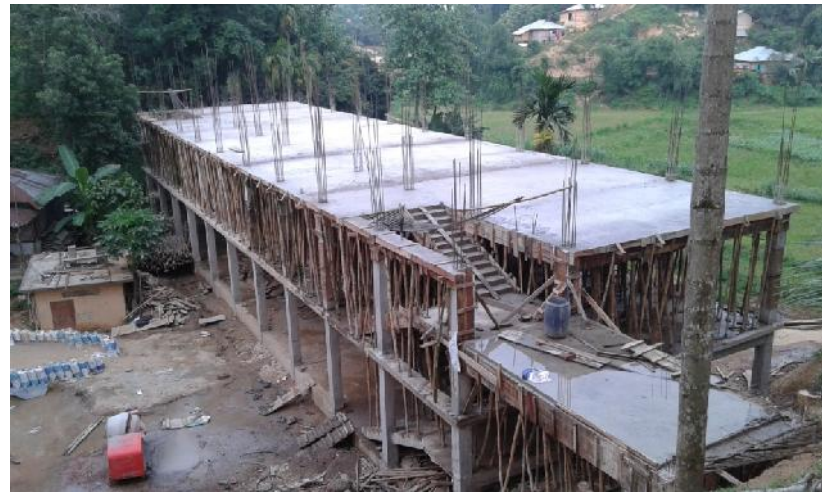
Plate 8: The 2 nd floor done!
