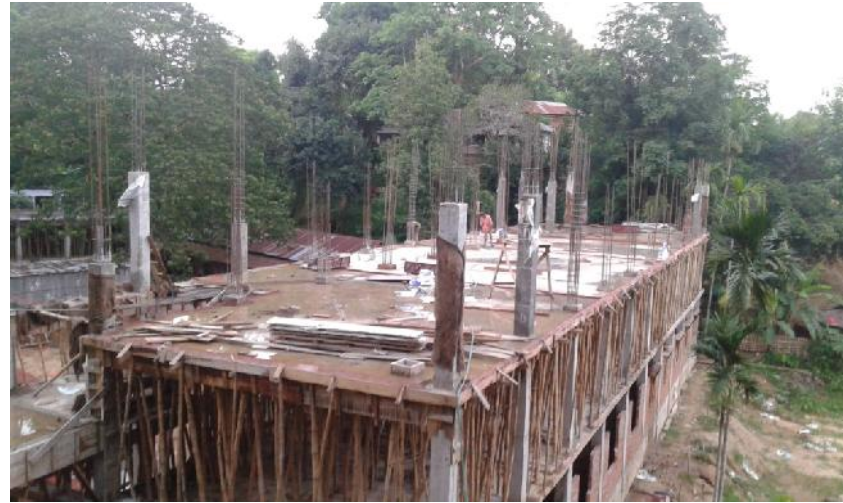
Plate 10: Putting up pillars for the 3 rd floor
