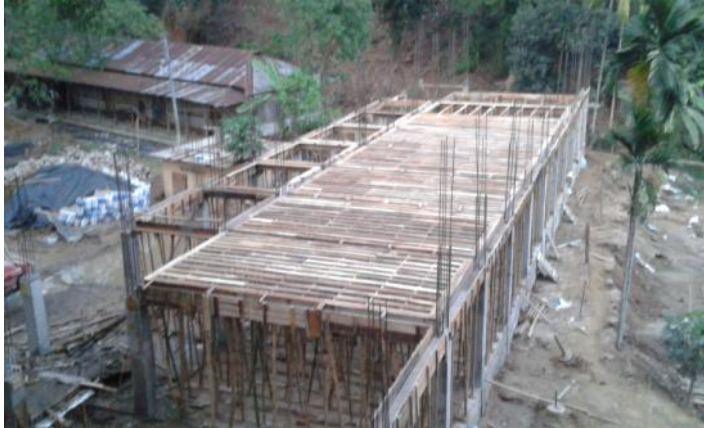
Plate 1: Preparation for the 1 st floor
