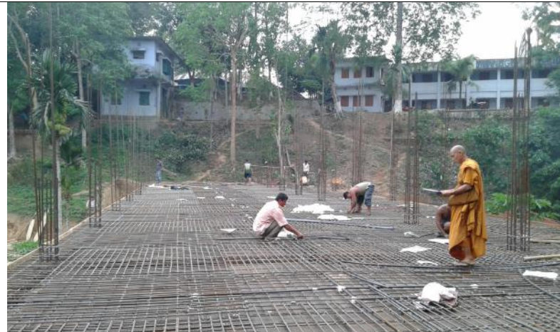
Plate 4: fixing pipes for electrical lines
