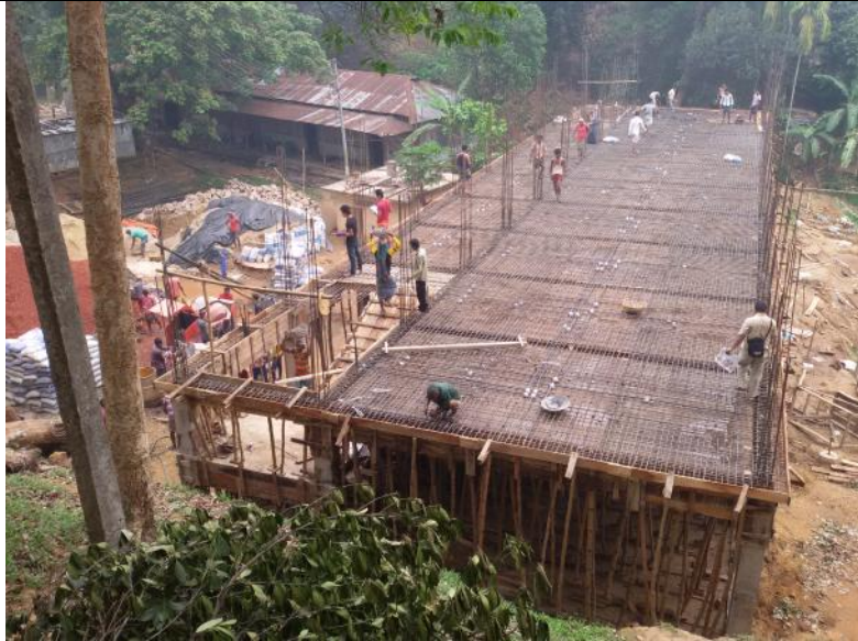
Plate 5: ready for casting
