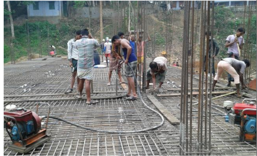
Plate 10: Casting on progress
