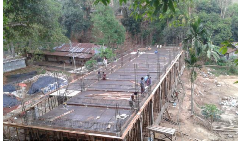
Plate 2: Preparation for the 1 st floor
