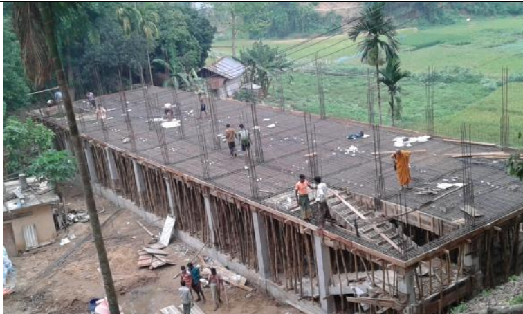
Plate 3: Fixing the iron rod for the 1 st floor
